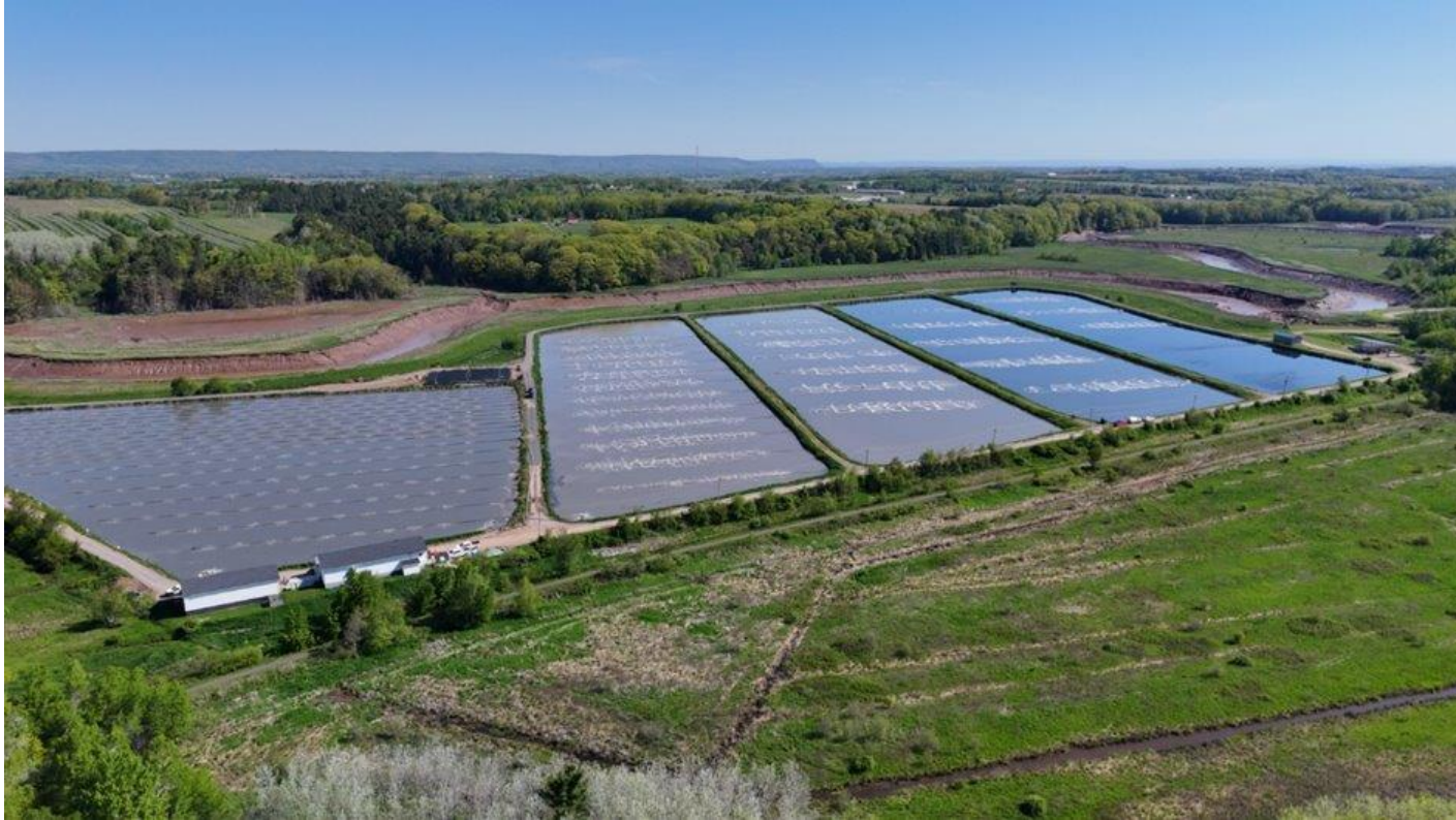
Regional Sewer Treatment Plant Aerial Photo, 2025
